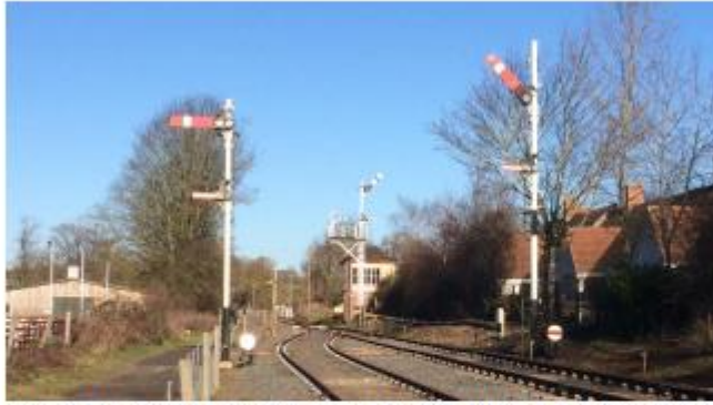
Image above: The trackwork and signalling installed at Boughton (looking north). The signal box was rescued from near Crewe. The Brampton Valley Way is to the left of the image, separated from the railway by a fence.
